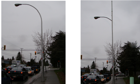
Figure 1: Example of the before (left) and after (right) attached telecommunication equipment. Adapted from Pilot Program for the Use of Street Light and Utility Poles for the Installation of Wireless Communications Infrastructure, by City of Surrey (2012). Retrieved February 27, 2014 from http://www.surrey.ca/bylawsandcouncillibrary/CR_2012-R186.pdf .
