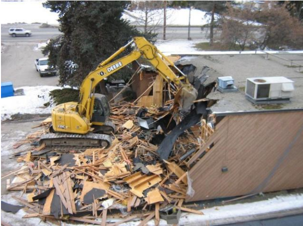
Old HQ demolition
