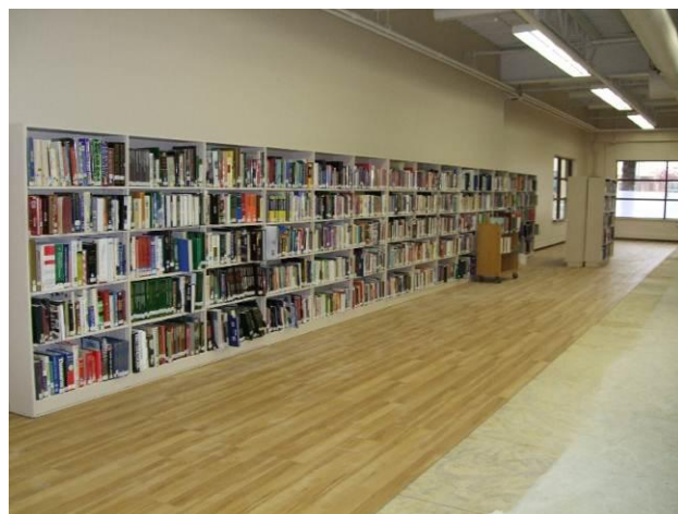
Early Progress in Flooring. Photo by TRPL Staff.
