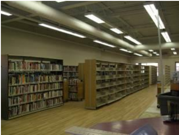
Flooring and Shelving in Progress. Photo by TRPL Staff.
