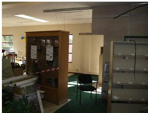
Office Wall, Half Removed. Photo by TRPL Staff.
