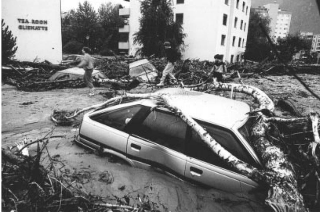
Figure 1. Car buried in mud after the devastating flash flood of the river Saltina in the town of Brig, Switzerland on 24 September 1993. (Photo: Coffrini, Sonntags Zeitung of 26 September 1993.)
