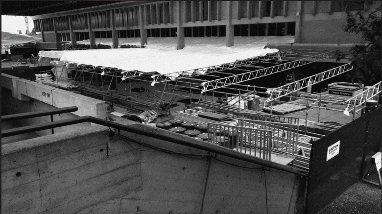
Building by Daniel Cheung
