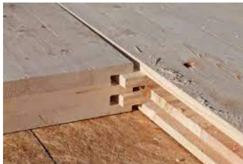
Figure 3: Interlocking Floor Joints Source: (Mohammad, 2011)
