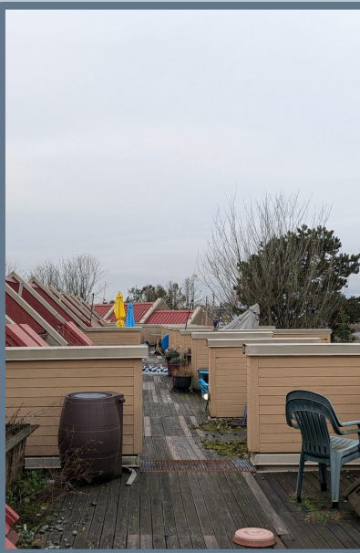
Figure 6. Shared Semi-Private Balcony Space
