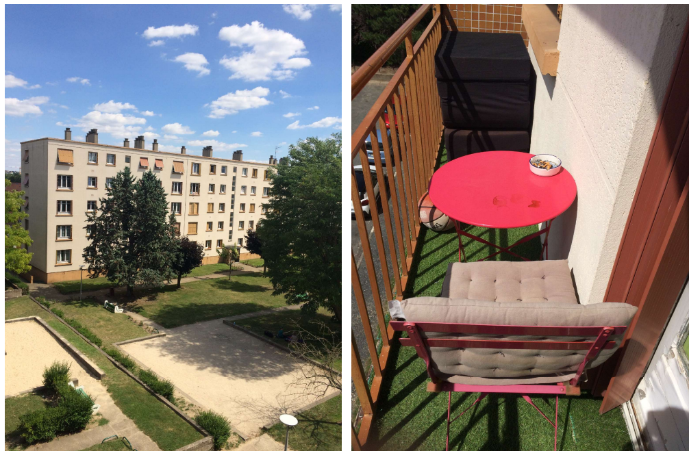
Figure 4. (a) Facade and common spaces of the building (b) balcony
